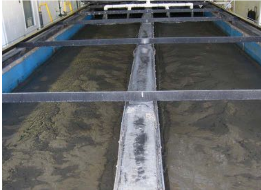
Thickened "TSS" is Inside the Container
