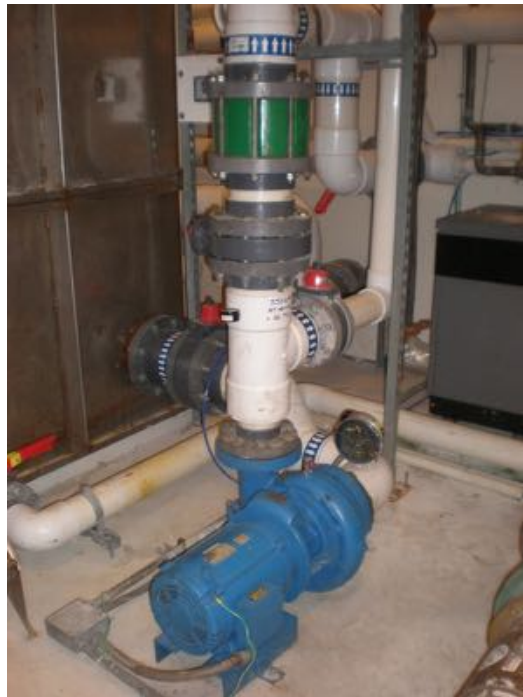
Pumps to Mix / Equalize the Tanks
