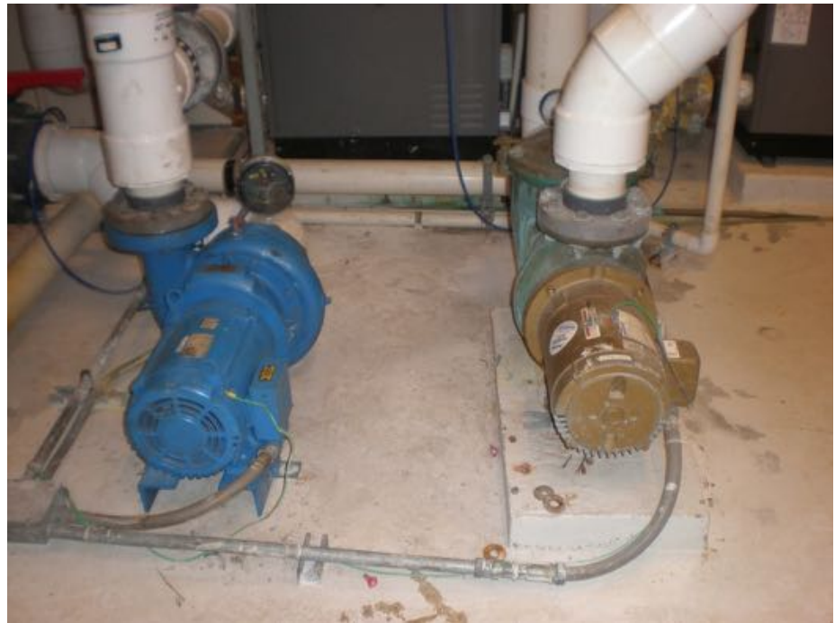
Pumps to Mix / Equalize the Tanks
