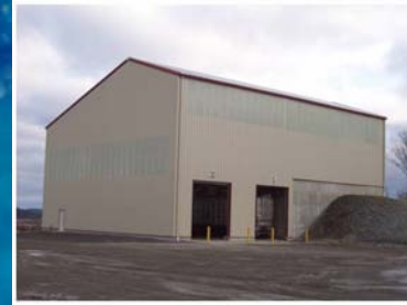
Door 19 Chute Door 20 Walking Floor Trailer Staging Area
