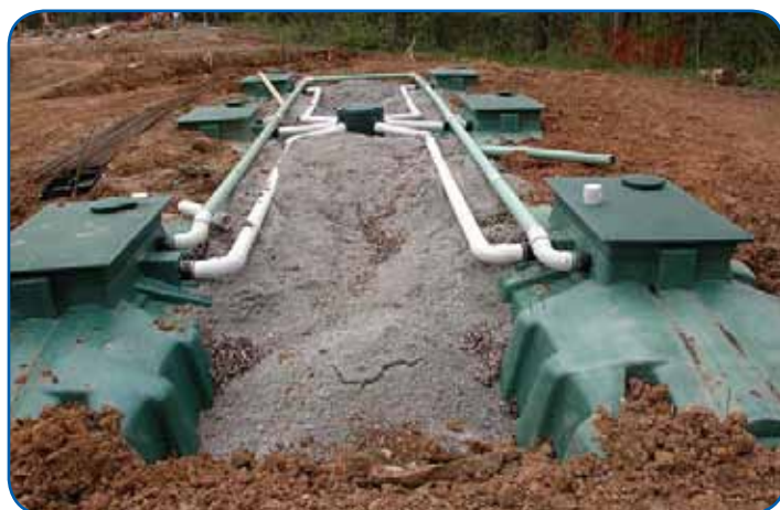
System for Visitor Center under construction. Courtesy of Bernheim Woods.
